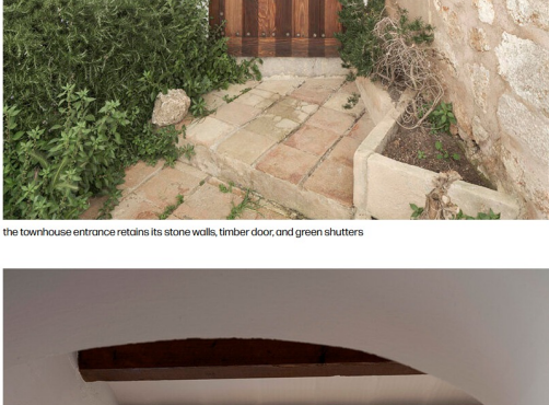
The restored townhouse sits within the stone houses and terraces of Banyalbufar
