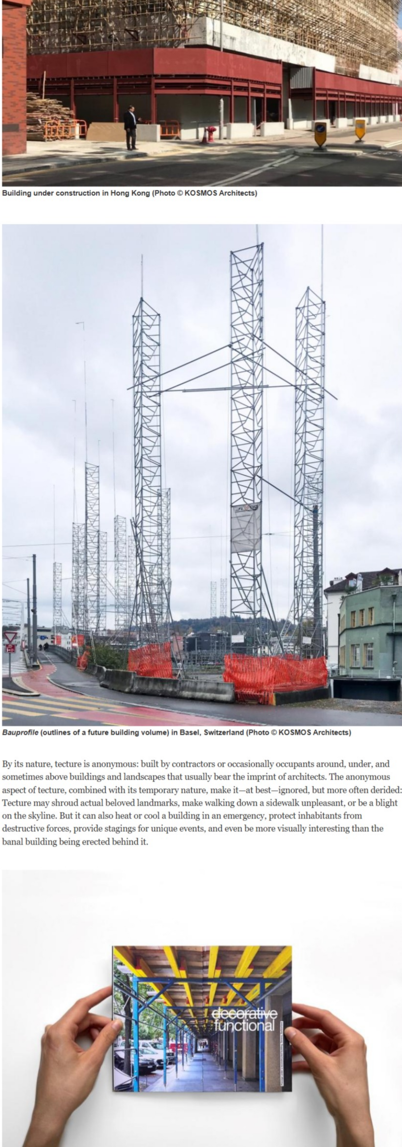
Building under construction in Hong Kong (Photo © KOSMOS Architects)
