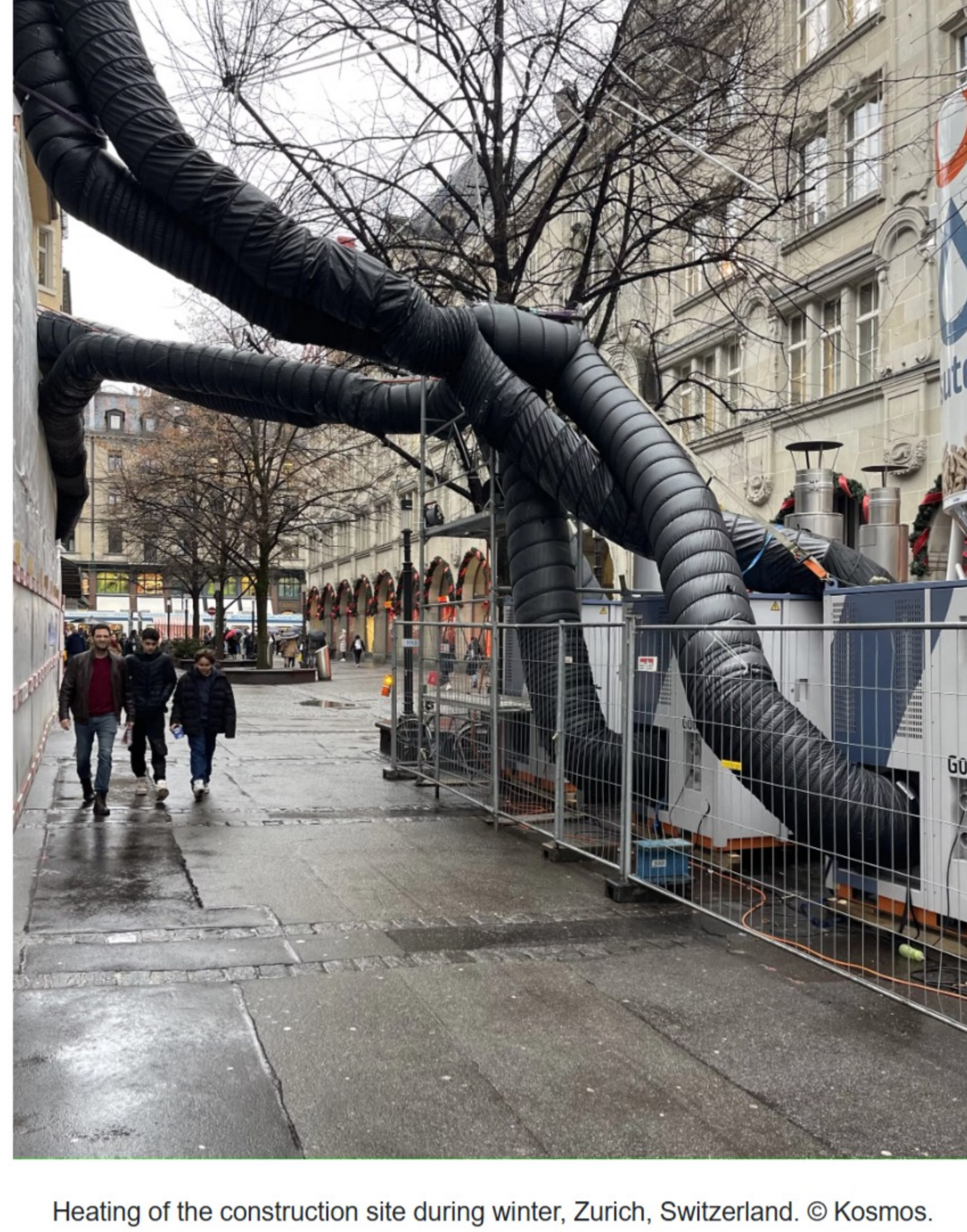
Heating of the construction site during winter, Zurich, Switzerland. © Kosmos.
